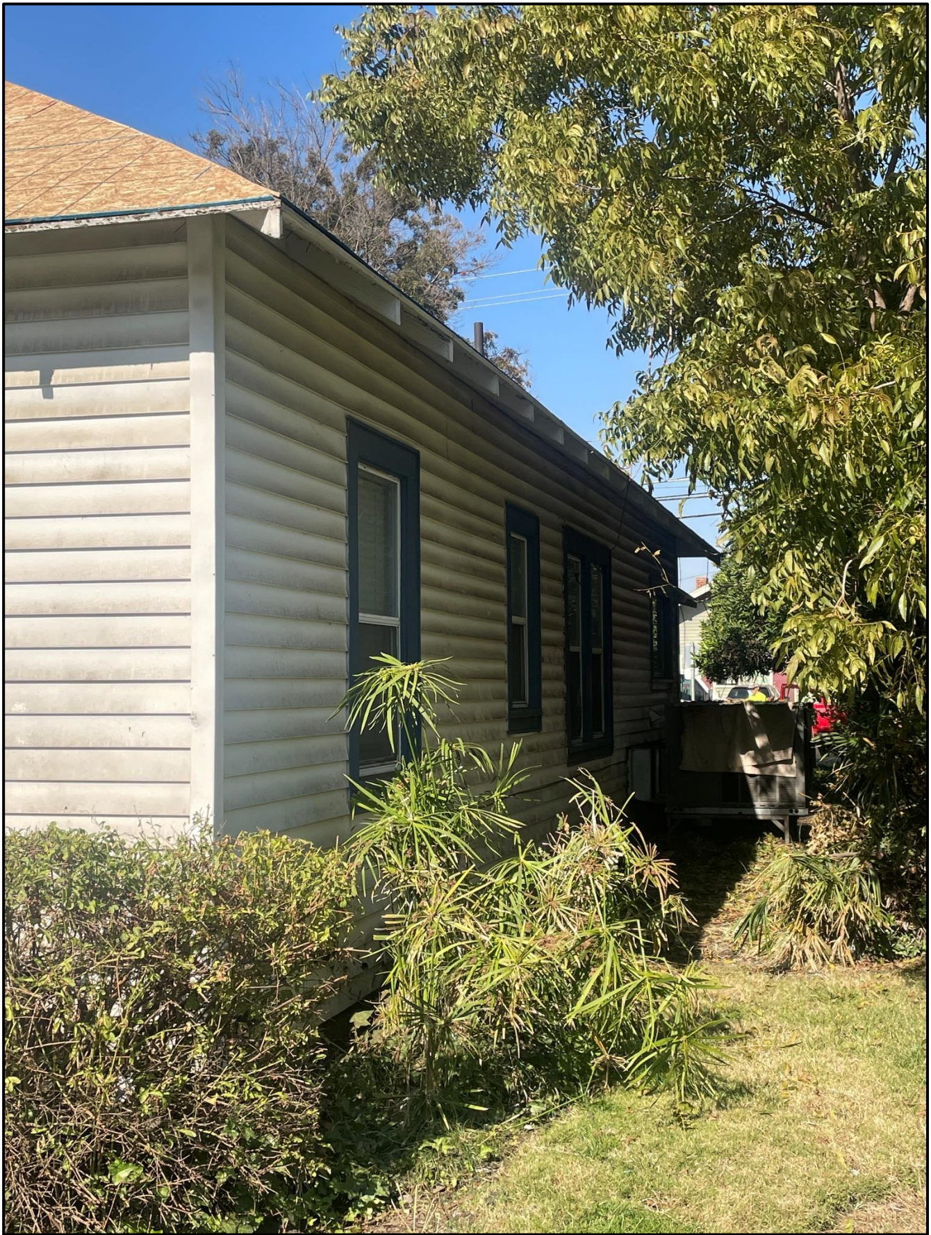
East Elevation – Facing 918 West Main Street
