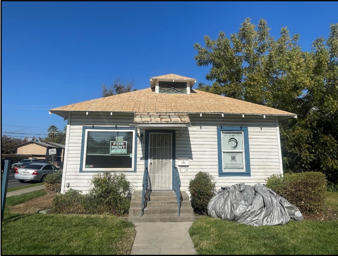
South Elevation – Facing West Main Street
