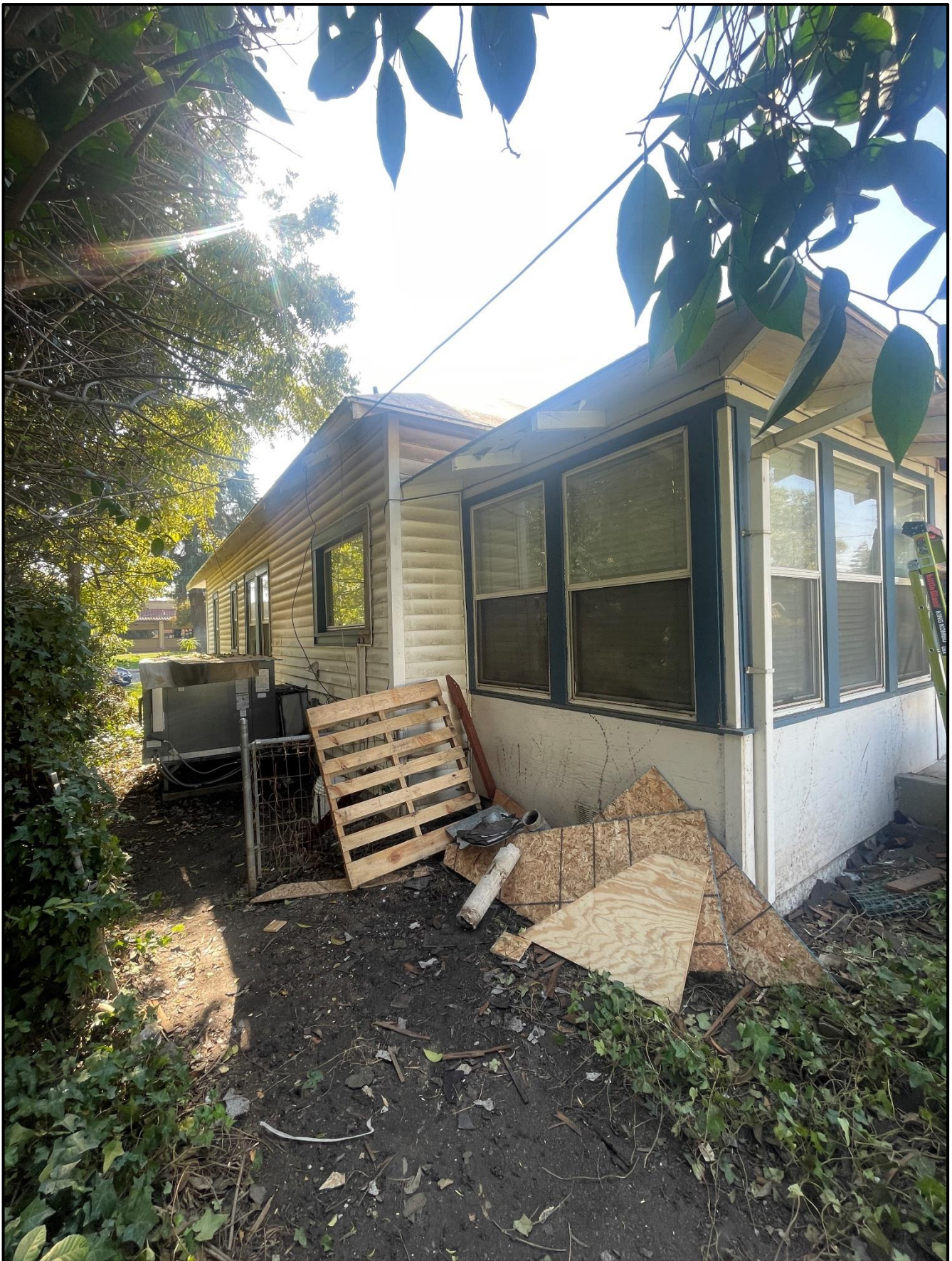
East Elevation – Facing 918 West Main Street
