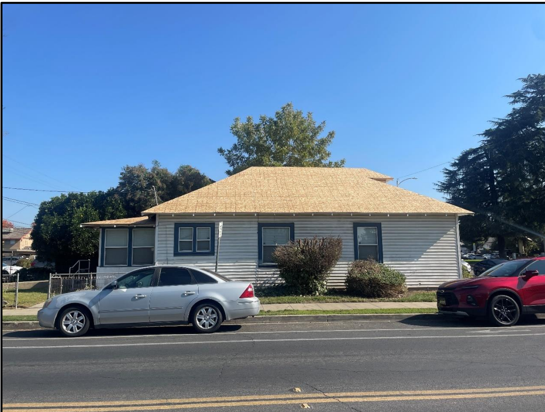
West Elevation – Facing North Jacob Street
