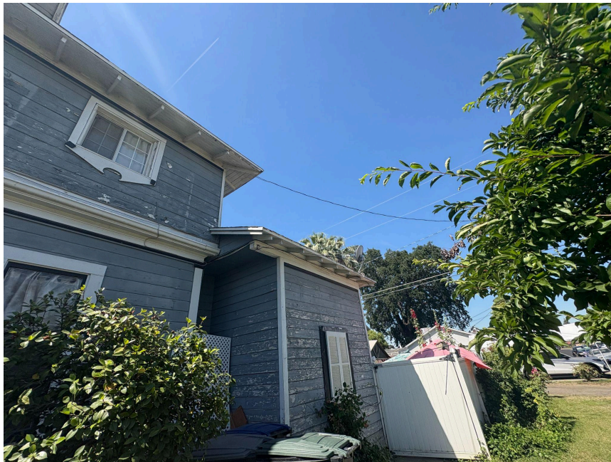
Rafter tails exposed, in decent condition, we would like to install fascia on all exposed rafter tails
