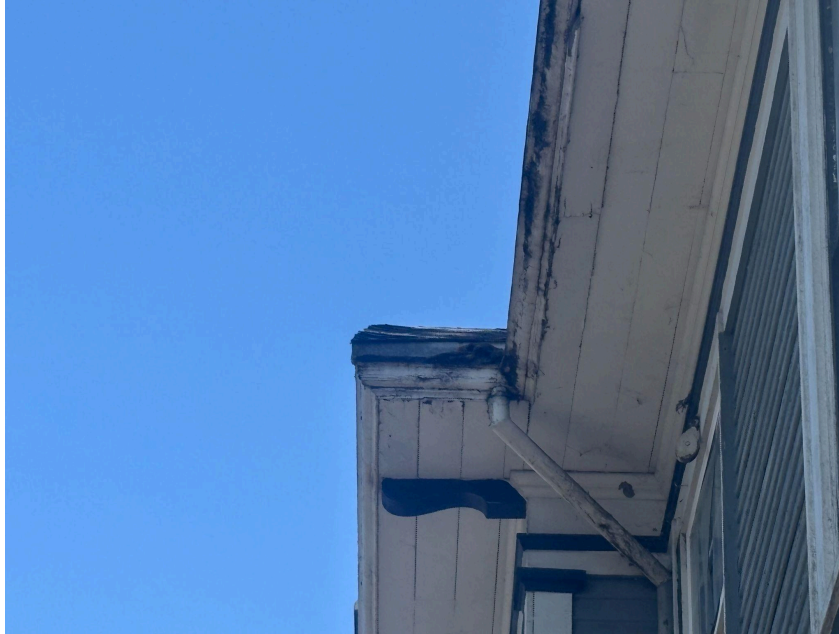
Evidence of wood rot in the original wooden gutter system, which has carried into fascia area
