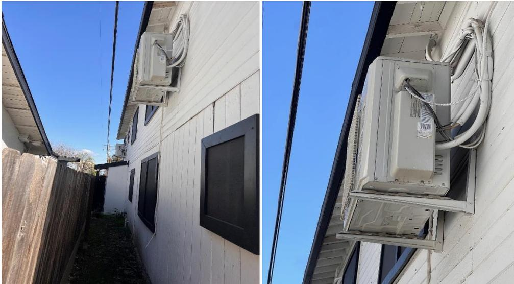
North Side of the Building: Remove/relocated HVAC (premature installation) to ground level. Will provide covering for wire, cables, lines, etc.
