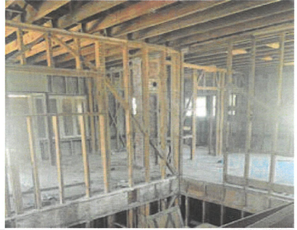
Exposed Bearing Wall System
