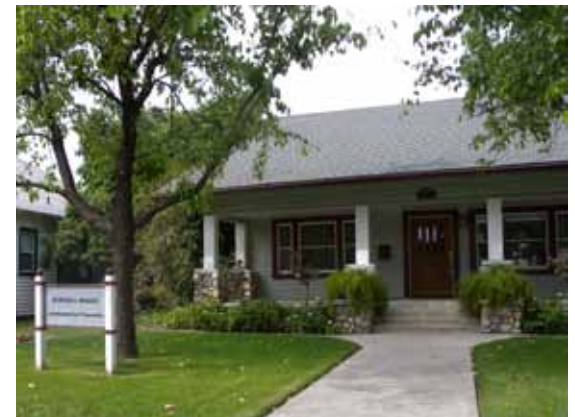
Preservation of some historic homes and buildings has been made possible with conversion to a new commercial or office use.
