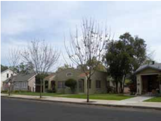
Property owners may use federal Historic tax credits or property tax abatement under the State's Mills Act program to help restore an historic house. (Top)
