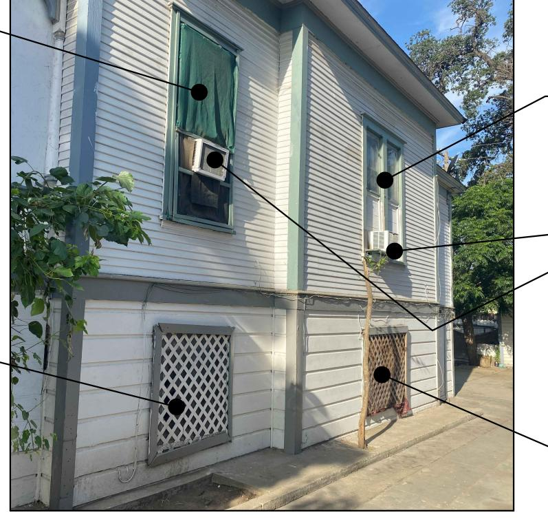
REMOVE (2) 2264 S.H. WOOD FRAME SINGLE PANE WINDOW AND REPLACE W/ NEW 2264 S.H. DUAL PANE, VINYL FRAME WINDOW.
