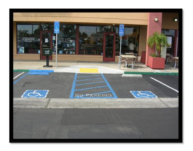
These parking stalls as illustrated, are code complying and accessible to persons with disabilities. They have all the elements of complying accessible parking stalls such as; width, depth, sign, ground marking, curb ramp, detectable warning, wheel stop, loading/unloading access aisle, and an accessible path of travel from the parking spaces to the entrances of small businesses in this strip mall.
